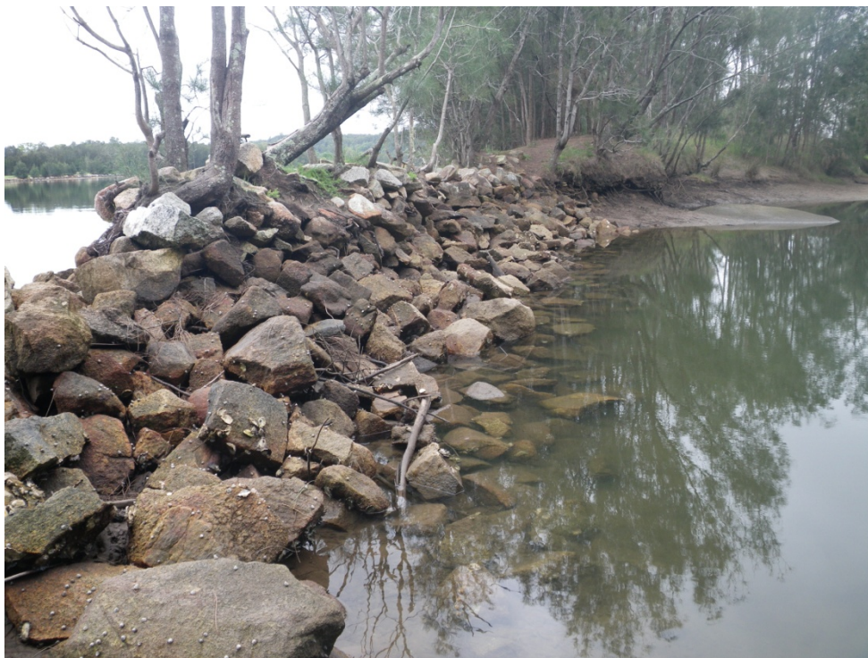
Figure 8: Man made rock wall constructed to retain the river bank, also traps fish on the outgoing tide.
